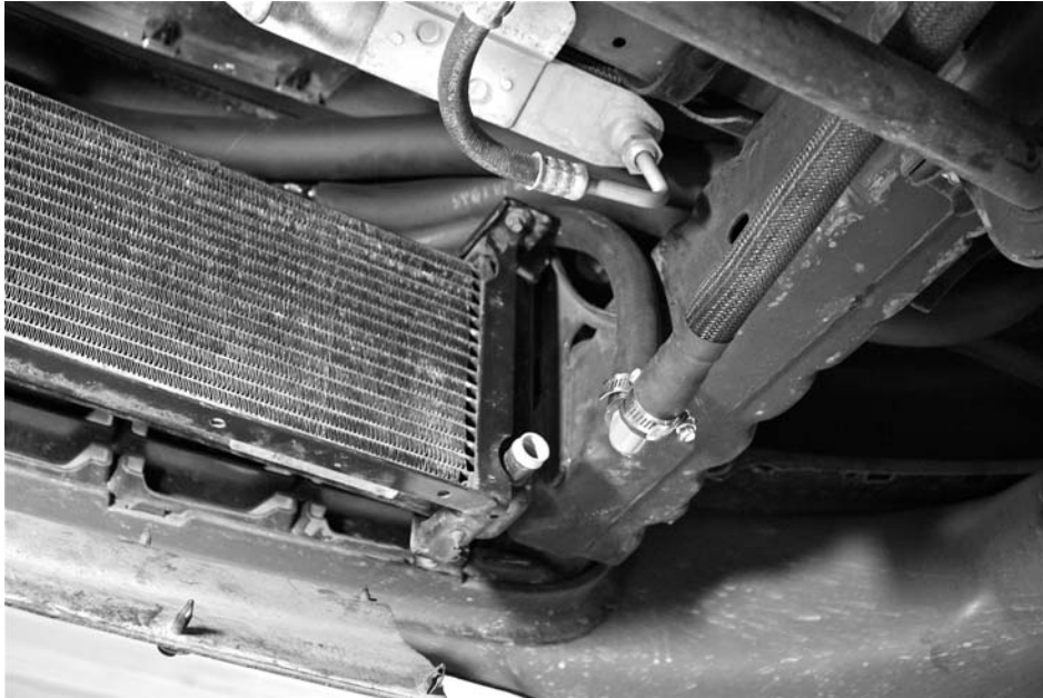
Photo showing steps 15, 16, and 17 completed.
